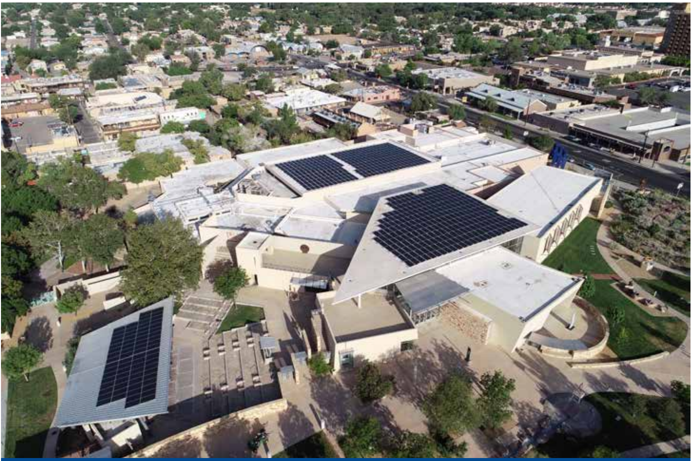
Rooftop solar panels on the Albuquerque Museum.
